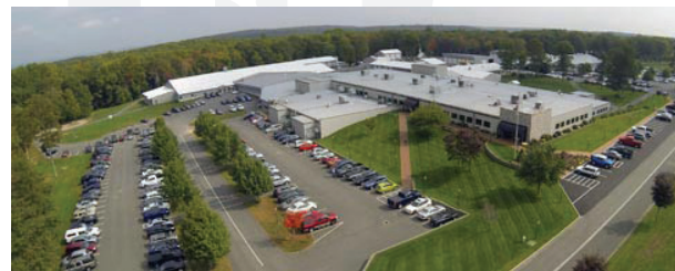
Chester, Connecticut facility
